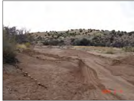
Fig. 4. Compound post vanes (set of three) slow water and force it to meander rightward and reconnect with the historic waterway.
