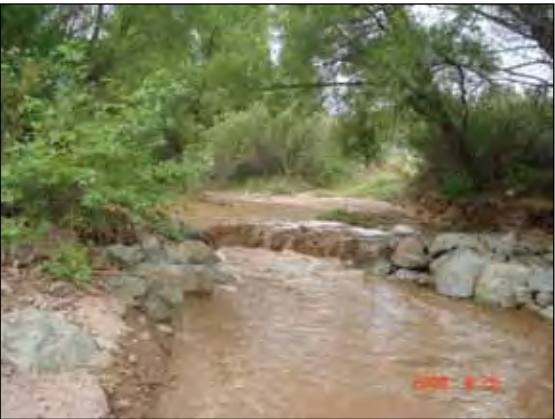
Fig. 2. Crossvane stabilizes cienaga by preventing headcut from eroding up cienaga.
