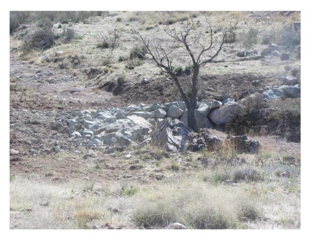
The photograph above is the same grade control structure immediately after construction and before rain. It is not common that a structure becomes completely "full" after only two rains, but in this case, the grade control structure captured the maximum amount of sediment that it is capable and a second tier atop the existing structure is necessary to continue reversing the erosive process that has been channelizing this drainage over the last century.
